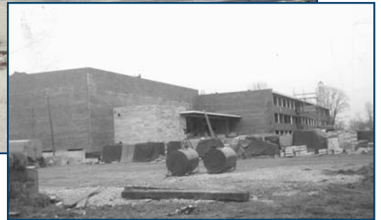
Construction of Bishop Chartrand, 1961
