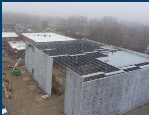
Gymnasium Construction Update
